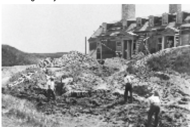
1934-35 Foundation Restoration, Officers' Quarters
