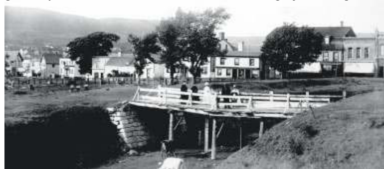
1895 Fort Anne Bridge
